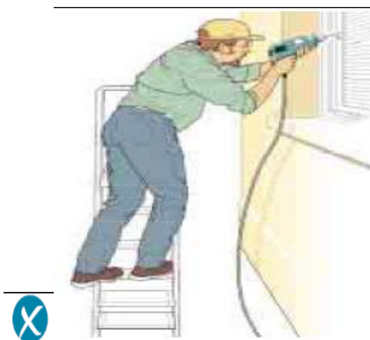
Incorrect – steps side on to work activity
